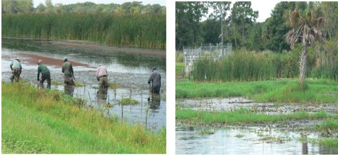
Figure 6. Bulrush planting in the northeastern portion Cell 2 (left) and transplants of alligator flag in the south end near outflow (right).
