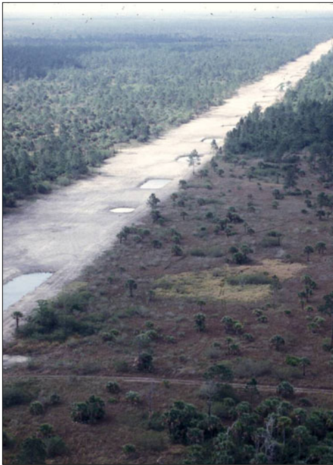
Figure 28. Prairie Canal after filling was completed.
