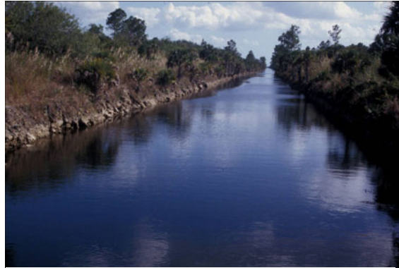
Figure 27. Prairie Canal prior to filling.
