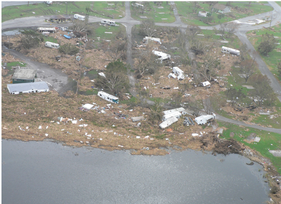
Figure 10-22. Damage to the Torrey Island Campground (photo by SFWMD).
