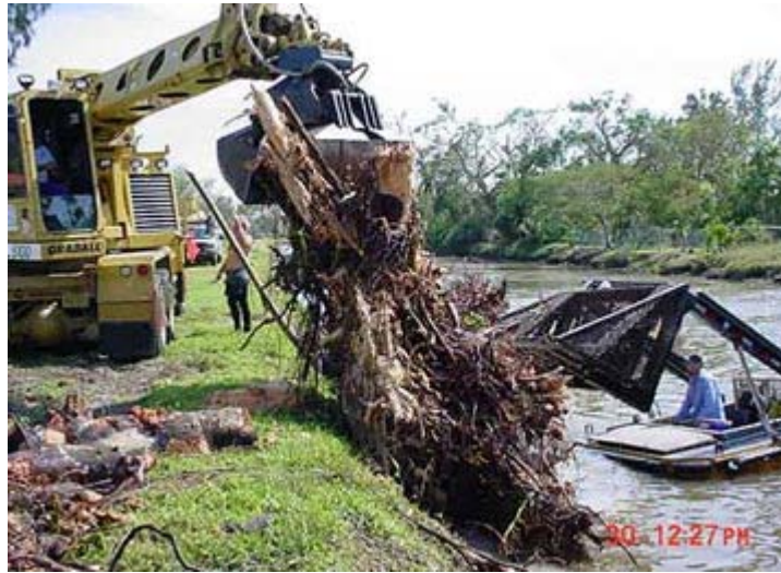
Figure 28. Removal operation of vegetation- and debris-filled canal after Hurricane Wilma (photo by SFWMD).
