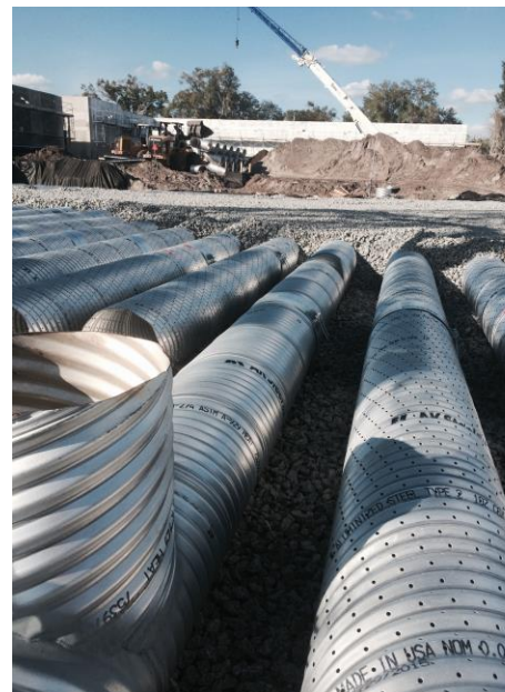
A typical containment row. Note the non-perforated row with full diameter cleanout access.
