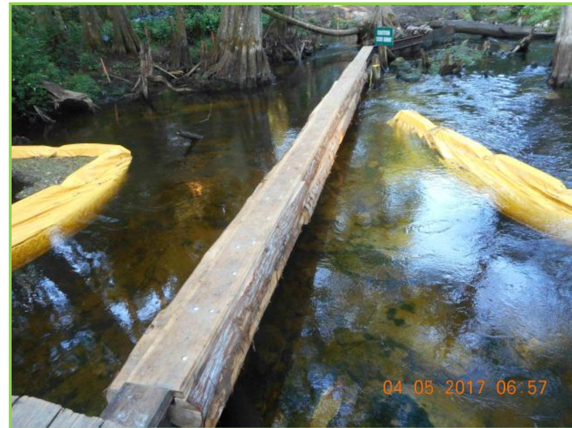
Cypress Logs being installed on the upstream side of dam
